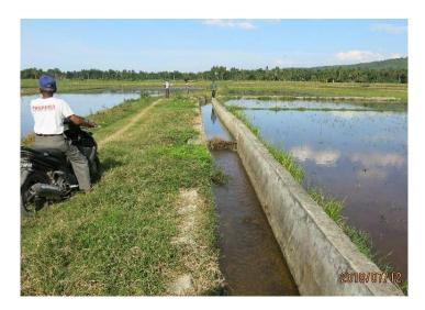
Irrigation canal in Manyang Lancok village with incomplete design and lack of maintenance. The canal is missing field gates. The community is not performing basic maintenance such and cleaning overgrowth. (World Bank, 2018)
